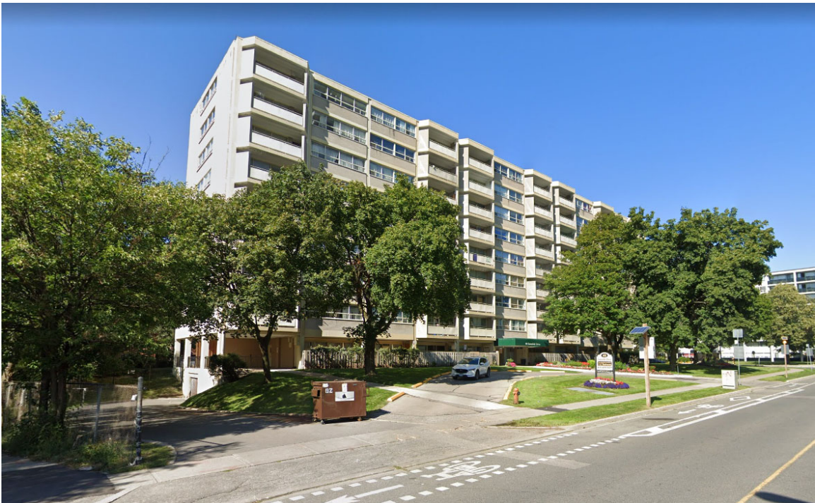
South West Corner along Grenoble Drive – Facing North East
